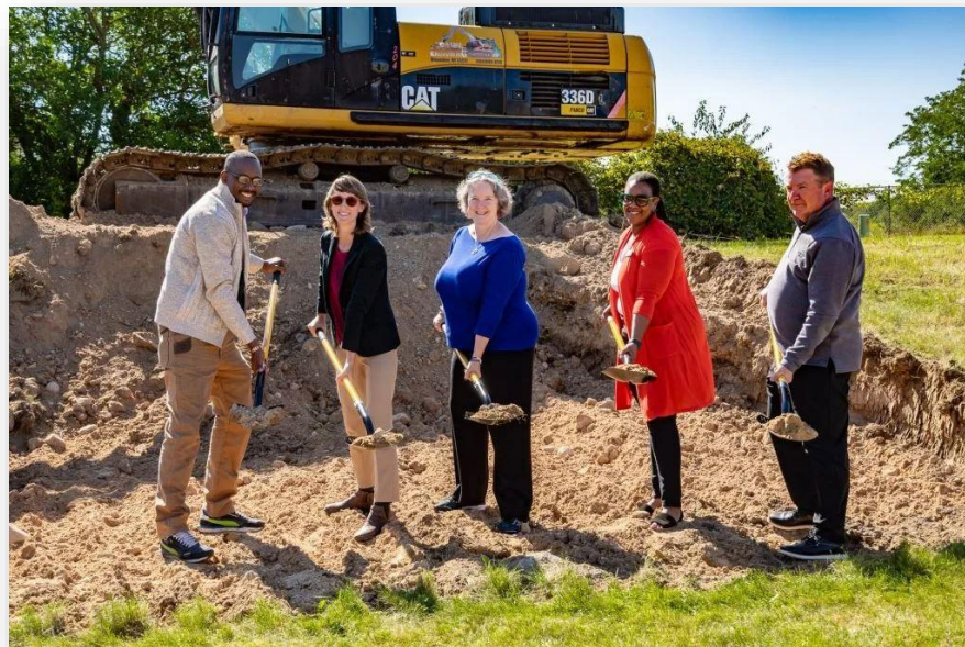
Groundbreaking on 4 new MACLT homes in Madison's Owl Creek neighborhood. Photo provided by MACLT.
